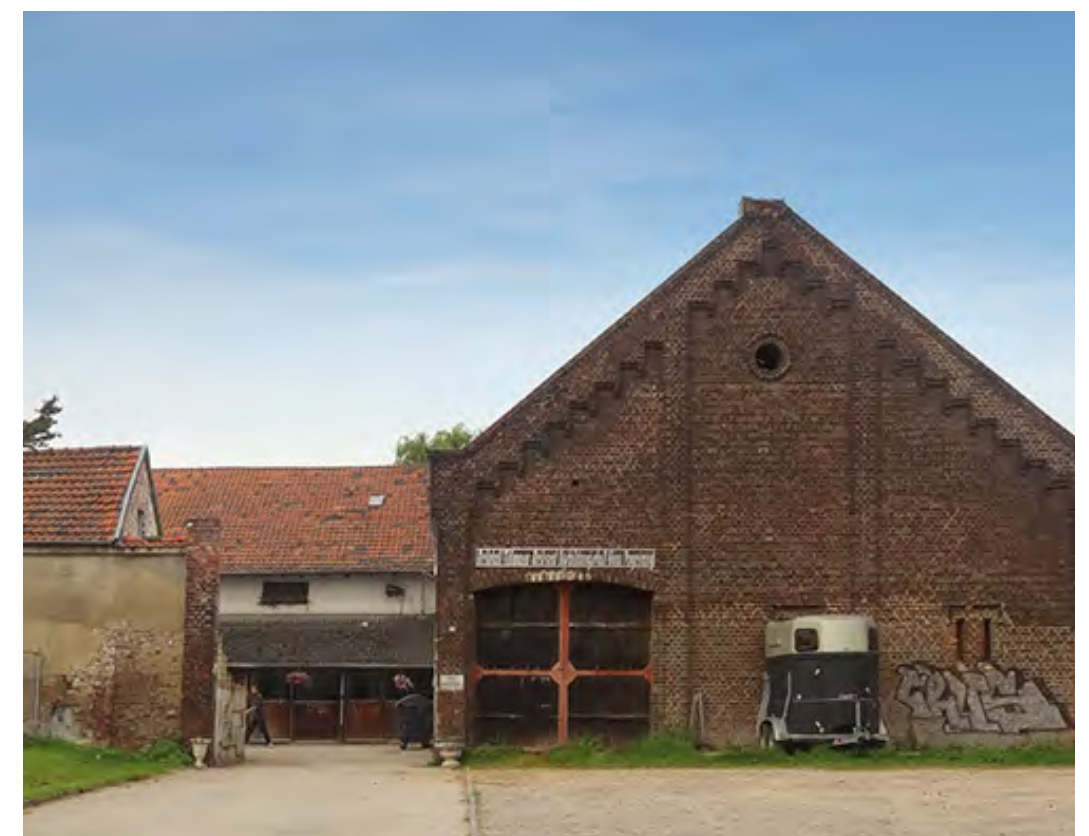
The remaining farm buildings shortly before demolition, 2016
